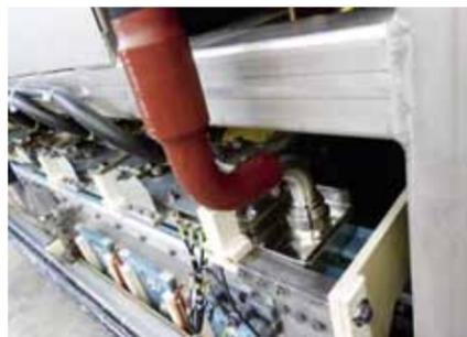
Special connecting ducts with 90° double bend, covered with shrink tubing sleeve for better electrical insulation
