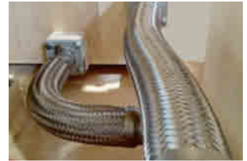
Flexible flow and return hose sections attached to the transformer.
