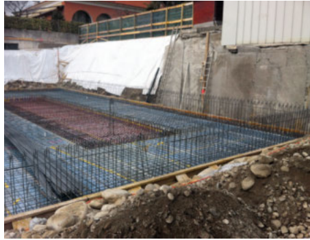
The right APSOPUR® antivibration mat for installation is selected according to surface pressure.
